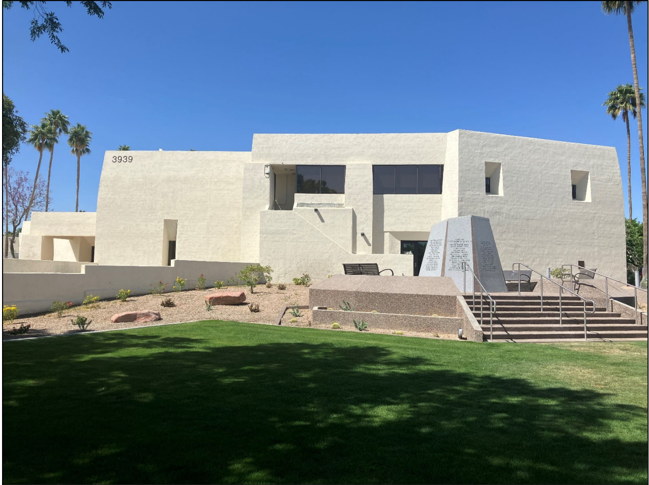
Photo 35. View of east elevation. View facing west (Logan Simpson, 2023)
