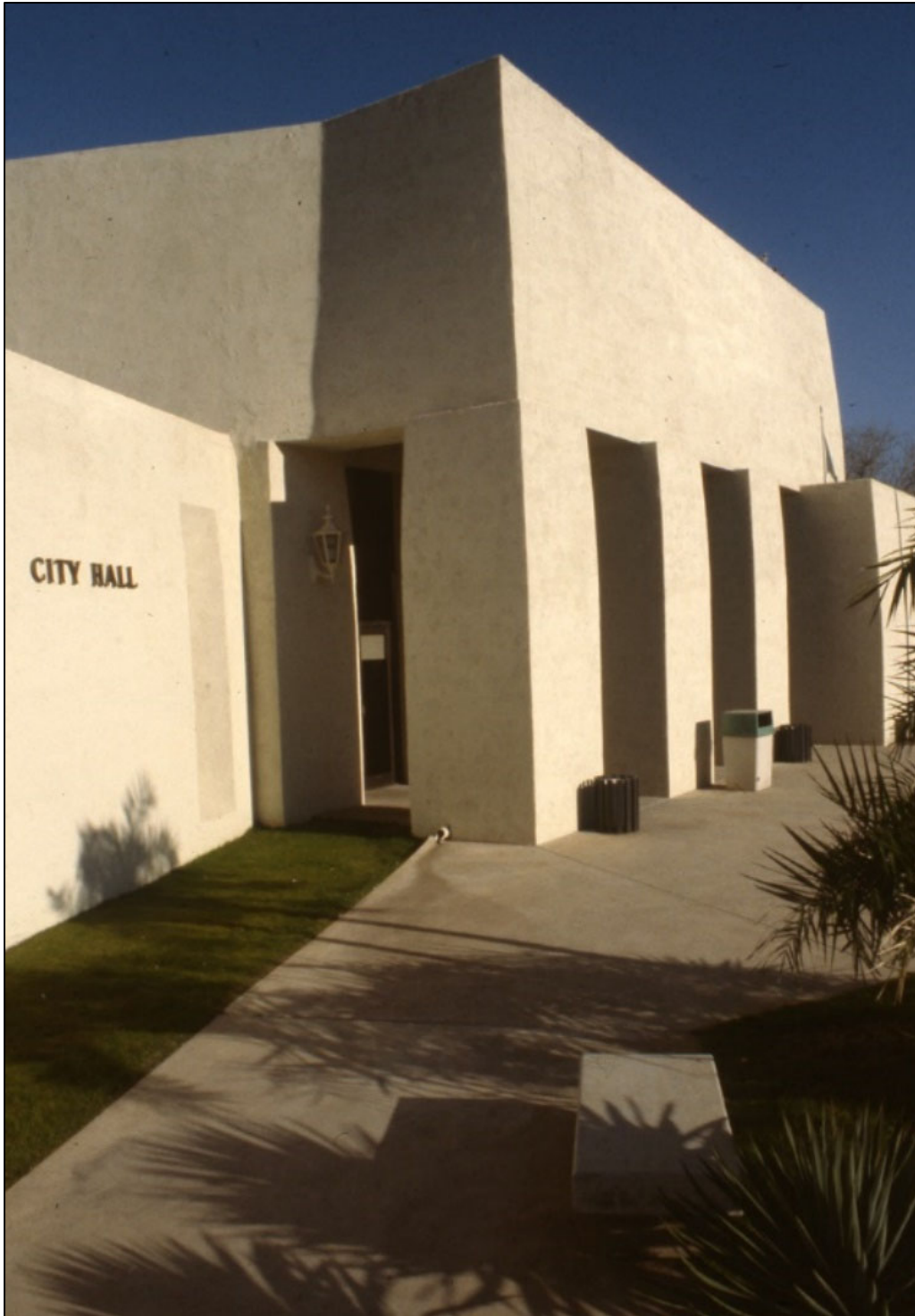
Photo 27. Historic view of the original entrance into Scottsdale City Hall, c. 1968 (Scottsdale Public Library)
