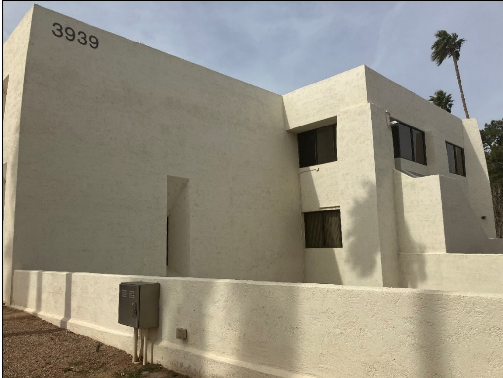
Photo 10. View of east elevation. View facing northwest (Logan Simpson, 2023)
