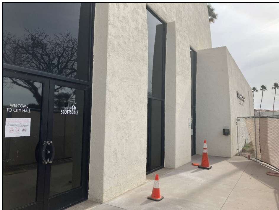
Photo 5. Entrance doors into Scottsdale City Hall. View facing southeast (Logan Simpson, 2023)
