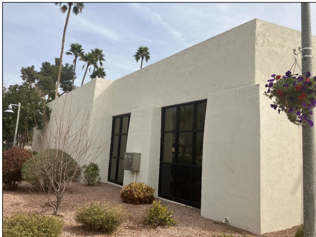
Photo 7. View of north elevation. View facing east (Logan Simpson, 2023)
