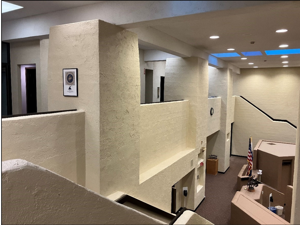
Photo 19. View of the mezzanine along the eastern wall. View facing southeast (Logan Simpson, 2023)
