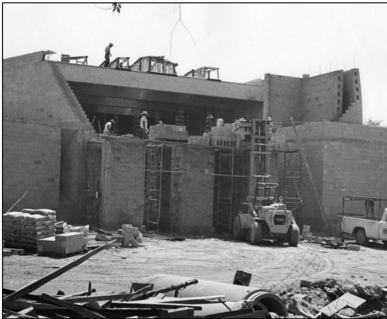
Photo 3. Historic view of the west elevation under construction. The double concrete block walls and beam construction can be clearly seen, c. 1967 (Scottsdale Public Library)
