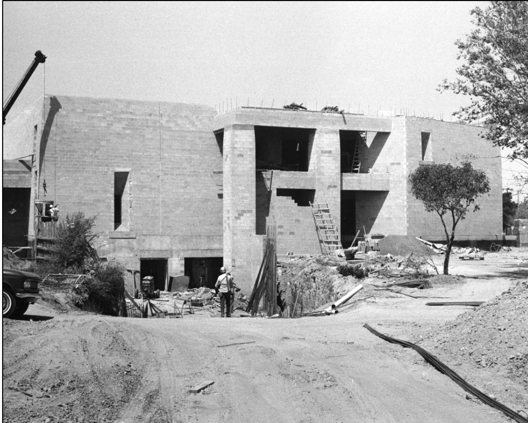
Photo 33. View of the east elevation under construction c. 1968 (Scottsdale Public Library)
