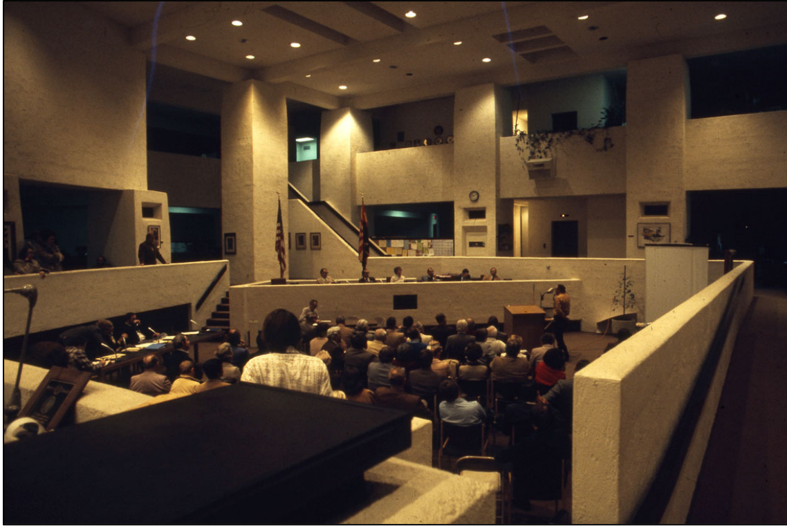
Photo 25. Historic view of the original dais, c. 1968 (Scottsdale Public Library)
