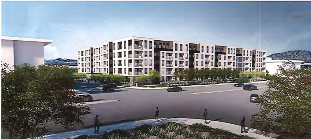
2 NE VIEW FROM RAINTREE DRIVE
