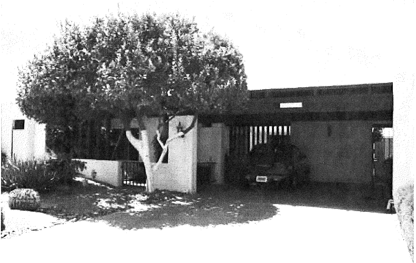
Lot 23, Type A1 - Wood post screen on stucco wall and wrought iron gate
