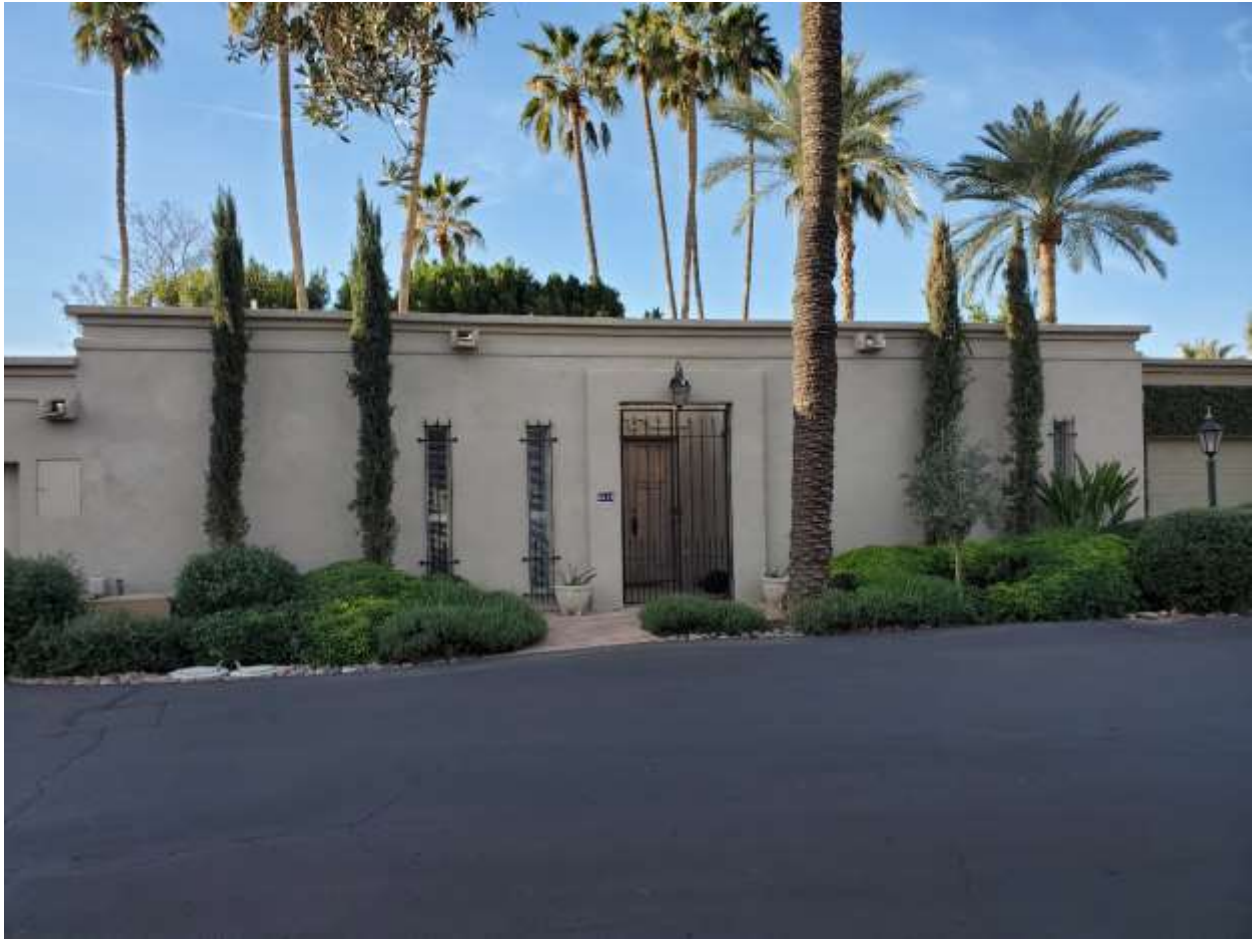
FIGURE 22 (NR Photo 13) One story unit, with original entry gates in place and the entry, and in front of the windows. The surface stucco texture is intact. .
