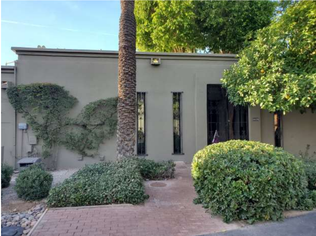
FIGURE 18 (NR Photo 9) One story unit with vertical windows and original façade texture and finish. The Entry gates are one of the original design options. Roofline is marked by the incised groove that was an original design option
