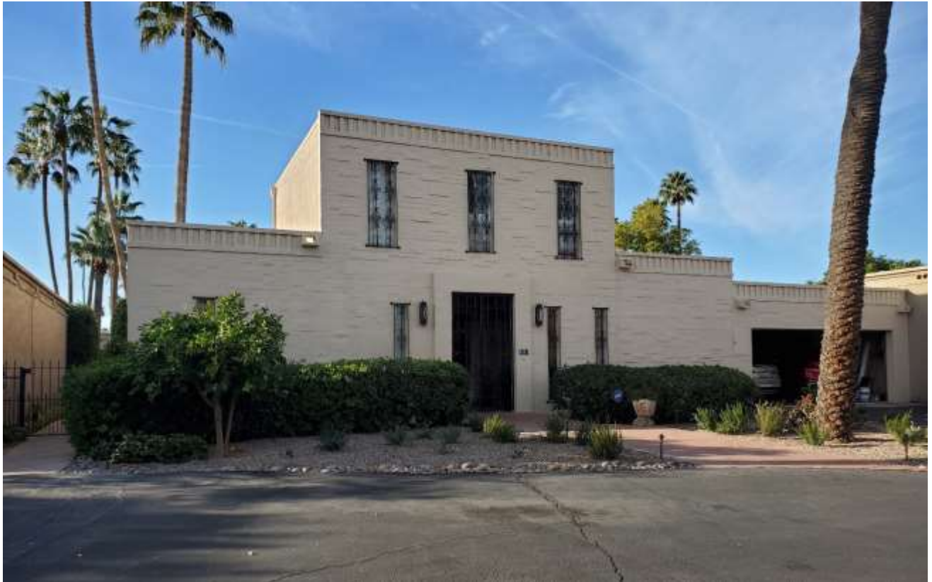
FIGURE 39 (NR Photo 30) Entry gates and surface texture are original. Typical two story unit with corbel detail at the roofline. Some of the two story plans have asymmetrical placement of windows on the first story depending on the location of the staircase, which varied with the floorplan.
