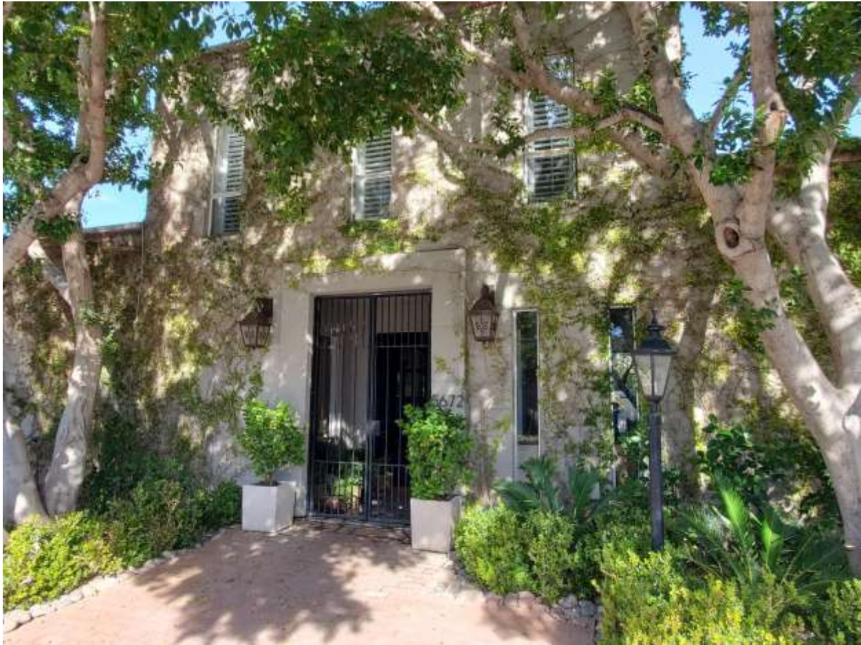
FIGURE 44 (NR Photo 35) Typical two story unit. Entry gates are original and the surface texture is original.
