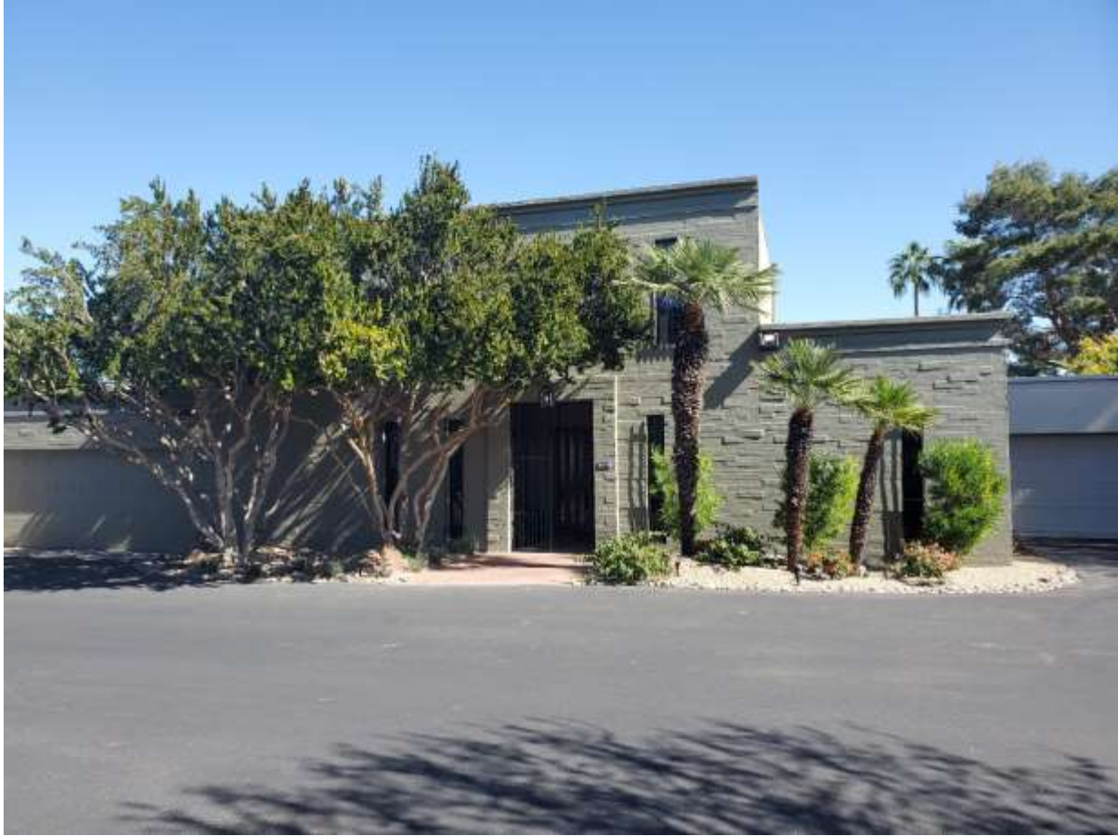
FIGURE 31 (NR Photo 22) 1Two story unit with original surface texture. Roofline highlighted by the corbel detail.
