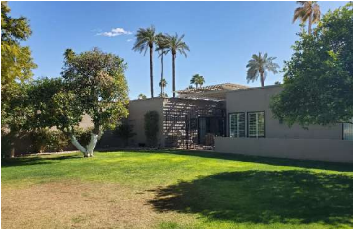
FIGURE 4 (NR Photo 43) Northwestern corner of courtyard, looking northwest. Unit has open atrium/patio with trellis shade structure which is the original condition for the units along the common space.
