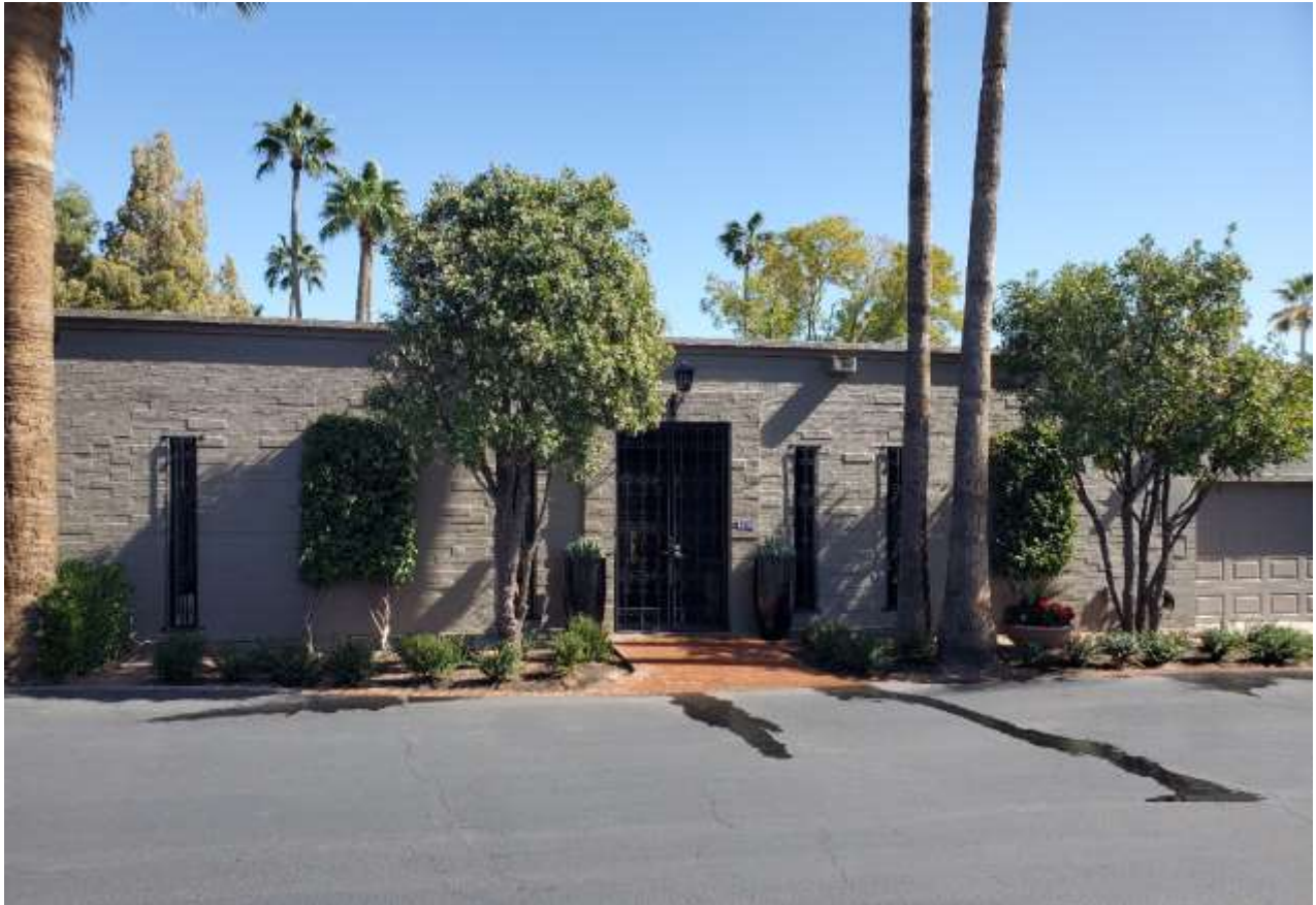
FIGURE 27 (NR Photo 18) Entry gates original. The surface texture is also original.
