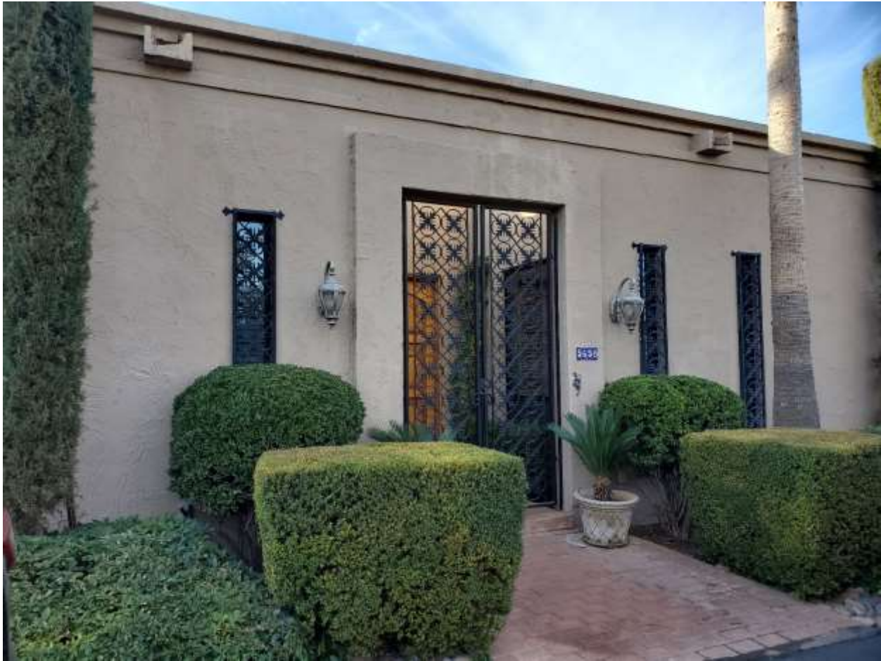
FIGURE 37 (NR Photo 28) Entry gates are original. The entry is recessed 8 feet. The surface texture has been altered but is consistent.
