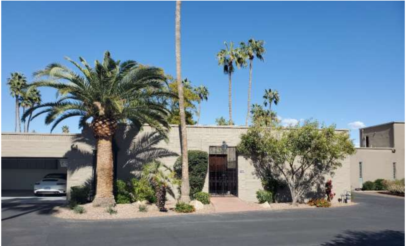
FIGURE 19 (NR Photo 10) One story unit that has the one of the original entry gate choices. The surface texture shows the option that emphasizes the projecting blocks, emulating the adobe tradition.
