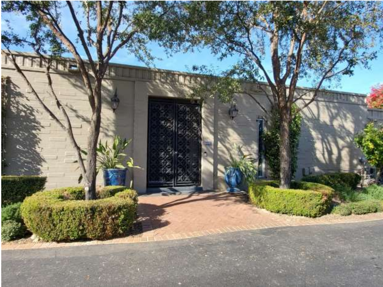
FIGURE 34 (NR Photo 25) Entry gates and doors are original. The surface texture is original. In this case the vertical windows on the left side of the entry are indicative of the floorplan. The roofline has the corbel detail.
