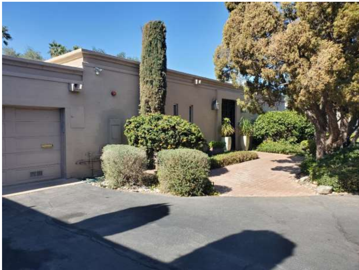
FIGURE 10 (NR Photo 1) Typical 1 story unit, accented by the recessed central entrance with a rectangular surround and wrought iron gate that is a replacement. There are two vertical windows on the south portion of the façade. The roofline is highlighted by a molded, corbelled cornice. The stucco now has a textured finish.
