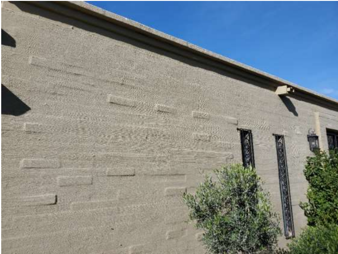
FIGURE 9: Primary stucco/wall "staggered block" texture with bricks projecting from wall plane in a random pattern suggesting adobe construction.
