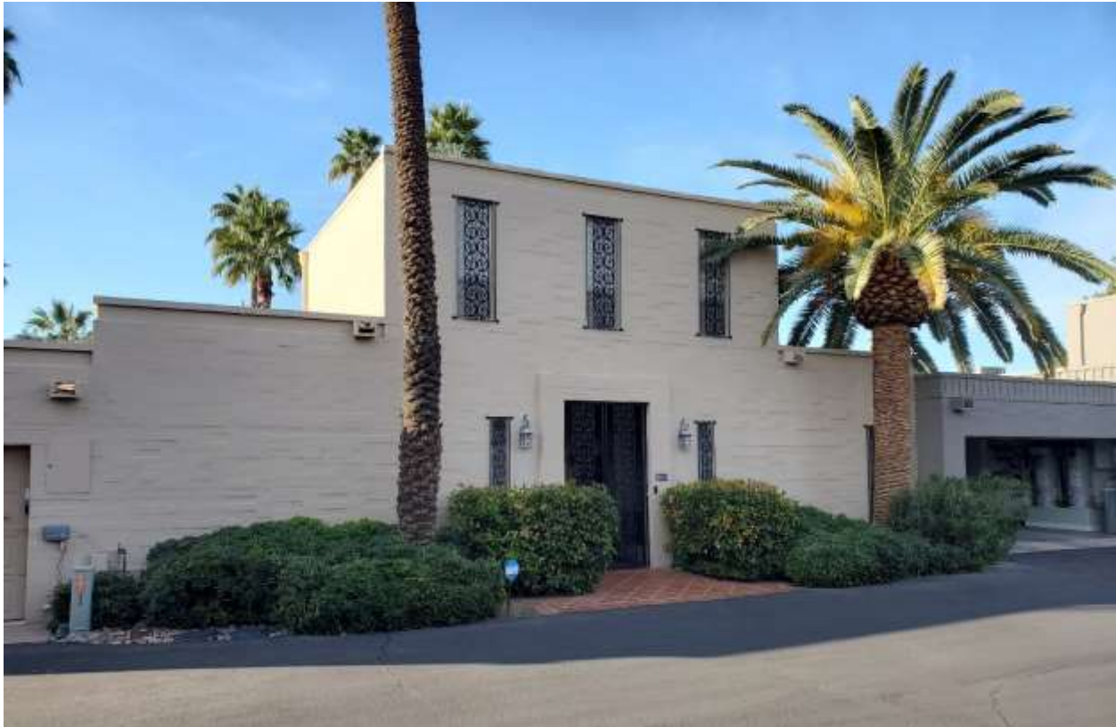
FIGURE 14 (NR Photo 5) Two story unit enhanced by overall symmetry. There are three windows on the upper story, symmetrically arranged over the central entrance below. The entrance is flanked by narrow vertical windows. All openings have matching iron grates. The façade surface shows the original texture and dimensionality. Entry gates are the original design.
