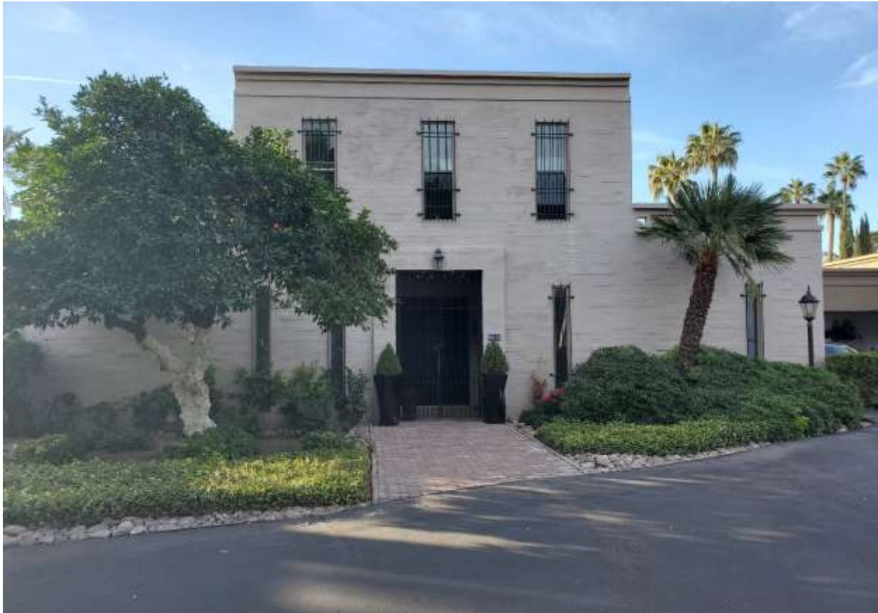
FIGURE 43 (NR Photo 34) The entry gates and surface texture are original and the roofline is a typical detail. In this case, the first story is symmetrical, corresponding to the internal floorplan.
