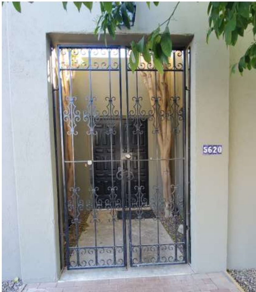
FIGURE 7 Typical example of original iron grates at the entrance. The gates are flush with the façade, and feature iron bars with varied curvilinear patterns. Depth of the foyer beyond the gates ranges from 3 to 8 feet, depending on the interior plan. Entrances to the larger units are shallower, entries to the smaller units are deeper.
