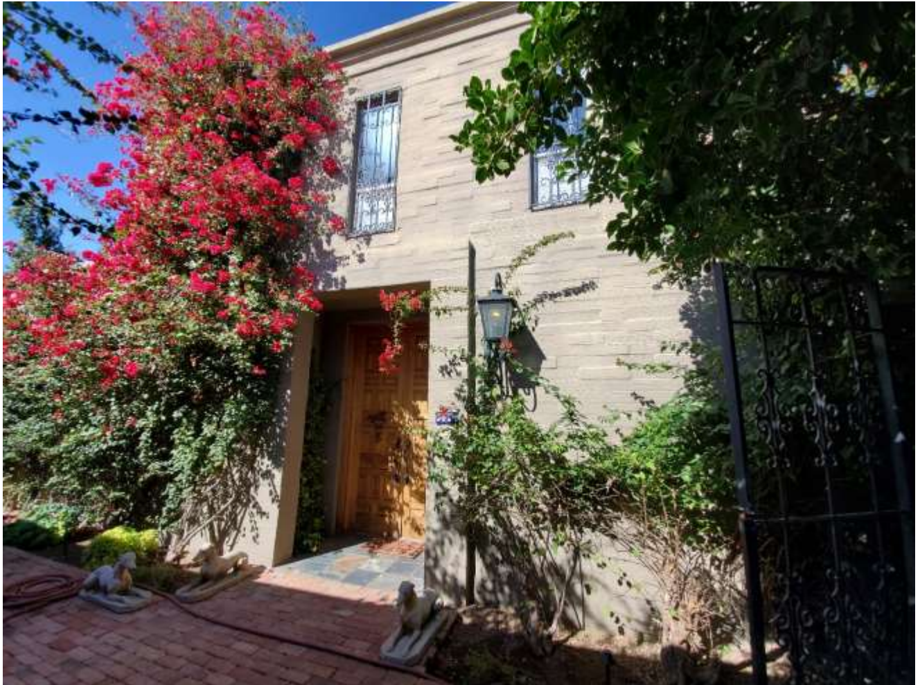
FIGURE 35 (NR Photo 26) Entry gates are original and the surface texture is original. The projecting cornice is one of the original design options.
