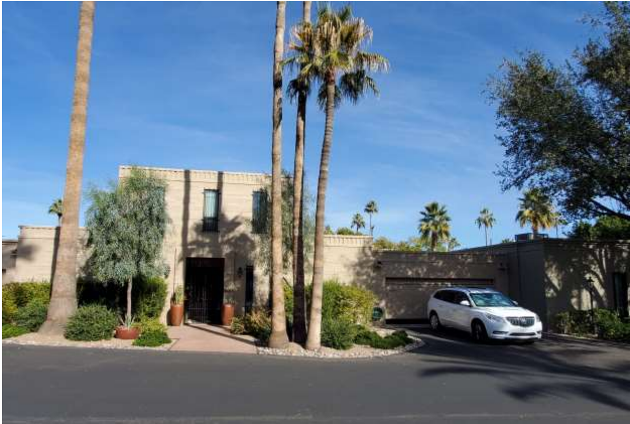
FIGURE 40 (NR Photo 31) Entry gates are an original design option. This is the two story design with corbel detail at the roofline.
