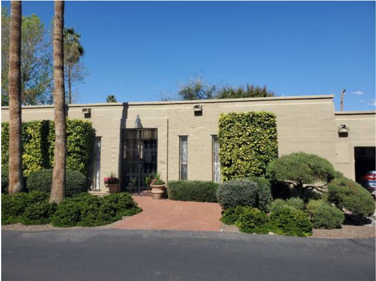
FIGURE 36 (NR Photo 27) Entry gates and the surface texture is original. Entry gates are original. Note the recessed groove at the roofline which is an original treatment. This unit has 4 vertical windows on the façade.
