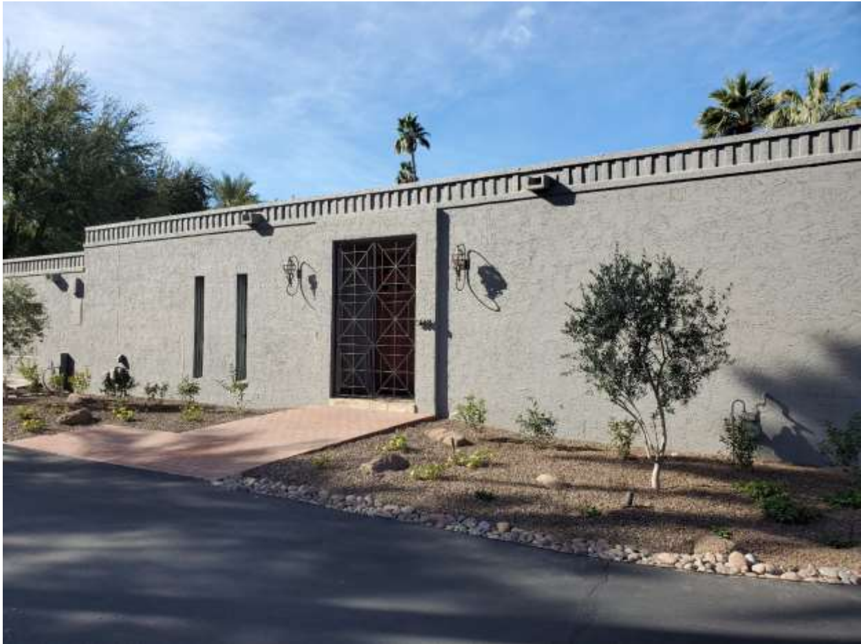
FIGURE 11 (NR Photo 2) One story unit with a central entrance. One of a few units that have been updated on the exterior, but the height and symmetry are intact. There are 2 vertical windows on the façade. The roofline is marked by a corbelled band which is a common detail. The façade surface is now textured stucco, not an original finish. The entry gate is a replacement design.
