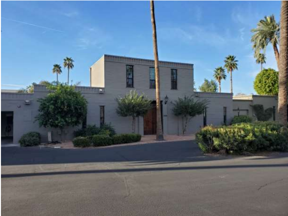
FIGURE 16 (NR Photo 7) Two story unit, three windows on the second story. Corbel table at roofline. Entry has rectangular surround. There are 5 vertical windows on the first level.
