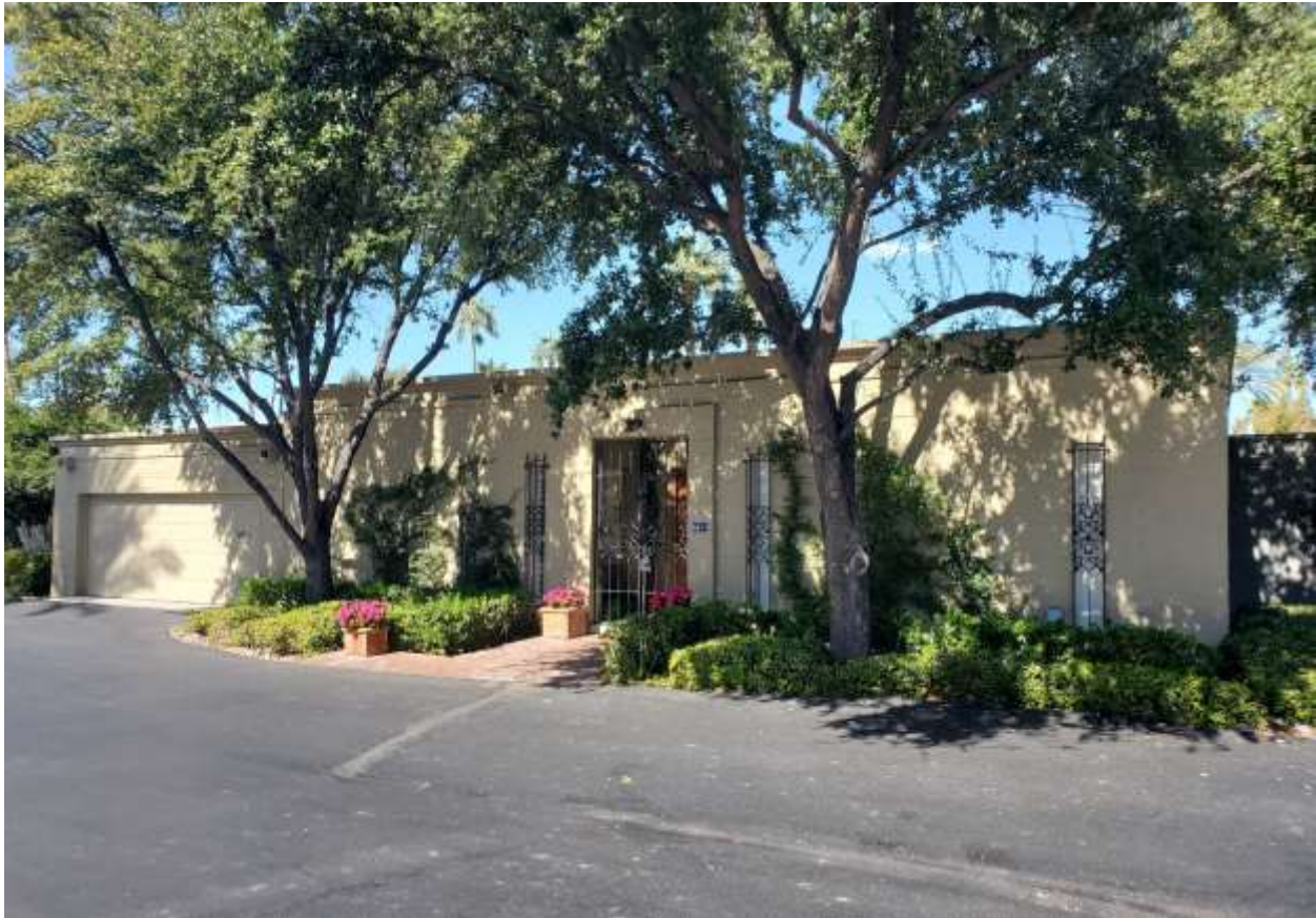
FIGURE 15 (NR Photo 6) One story unit with central entrance framed by heavy molded surround. There are five vertical windows. The entry door and windows have matching wrought-iron gates. The roofline features a molded cornice. The surface shows the original, undulating texture.
