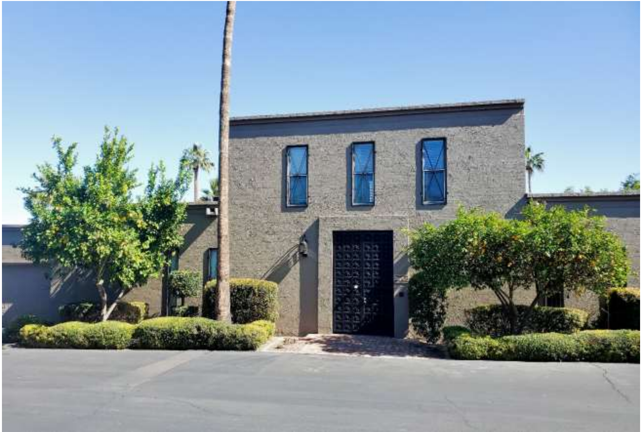
FIGURE 33 (NR Photo 24) Typical 2 story unit. Original surface texture.
