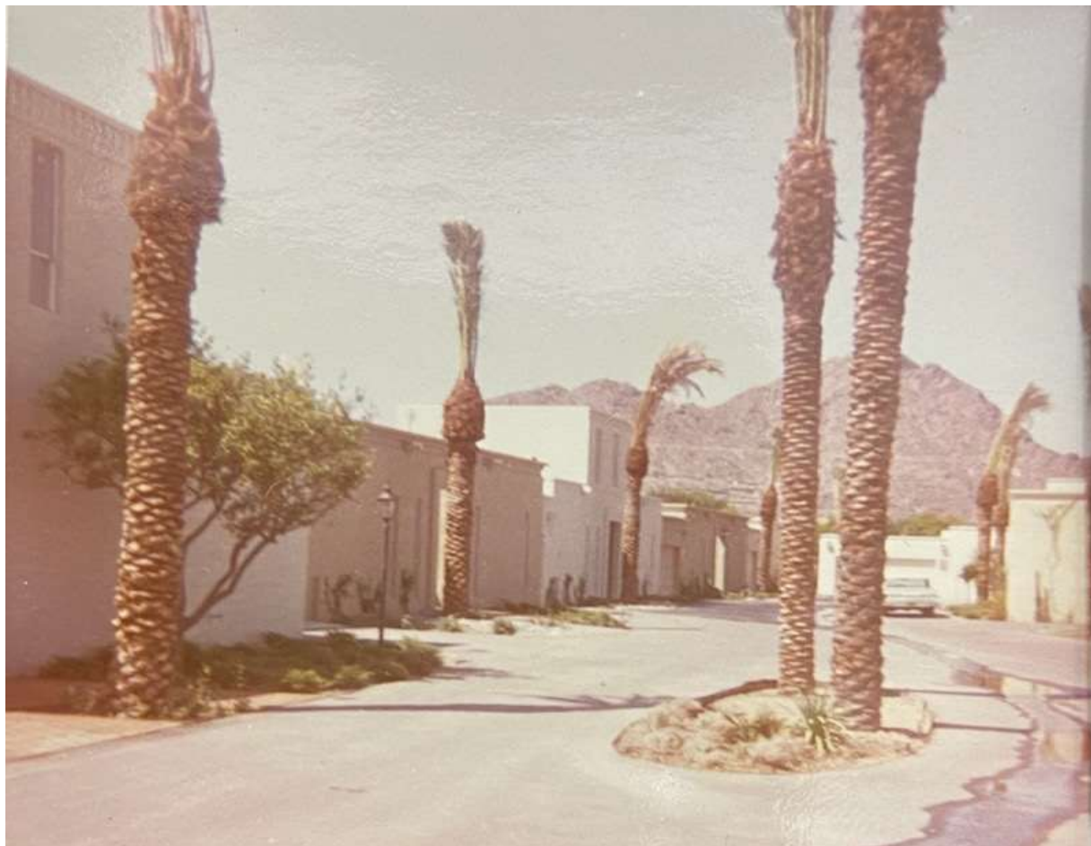
FIGURE 6 Looking north along western section of street at completion of construction, 1969. Trees and plants had been recently planted by developer. Photo from Stenjem family archives.
