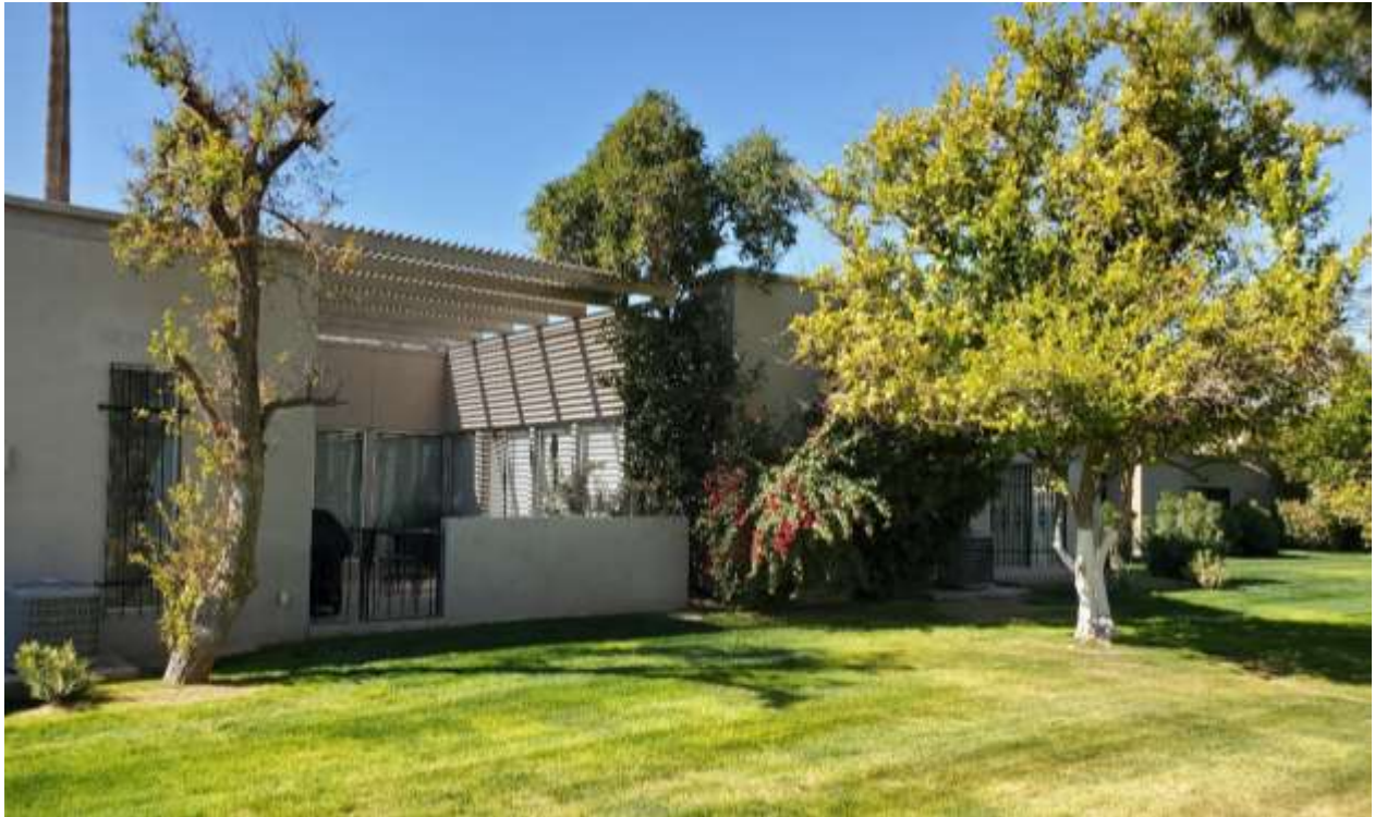
FIGURE 5: (NR Photo 44) Southwestern corner of courtyard, looking west. Unit has open atrium/patio with trellis shade structure which is the original condition for the units along the common space. The trellis over the patio is original although there are variations of the shade structures on other units.
