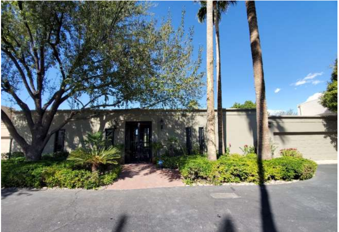
FIGURE 42 (NR Photo 33) Typical one story unit with five vertical windows. This house shows a slight modification in the window width on the left side to allow that bedroom to meet current City of Scottsdale code for egress. The windows on the right side are original. Of special interest, this unit was occupied by the developers, Elden and Weme Stenjem at the time Scottsdale North was completed.
