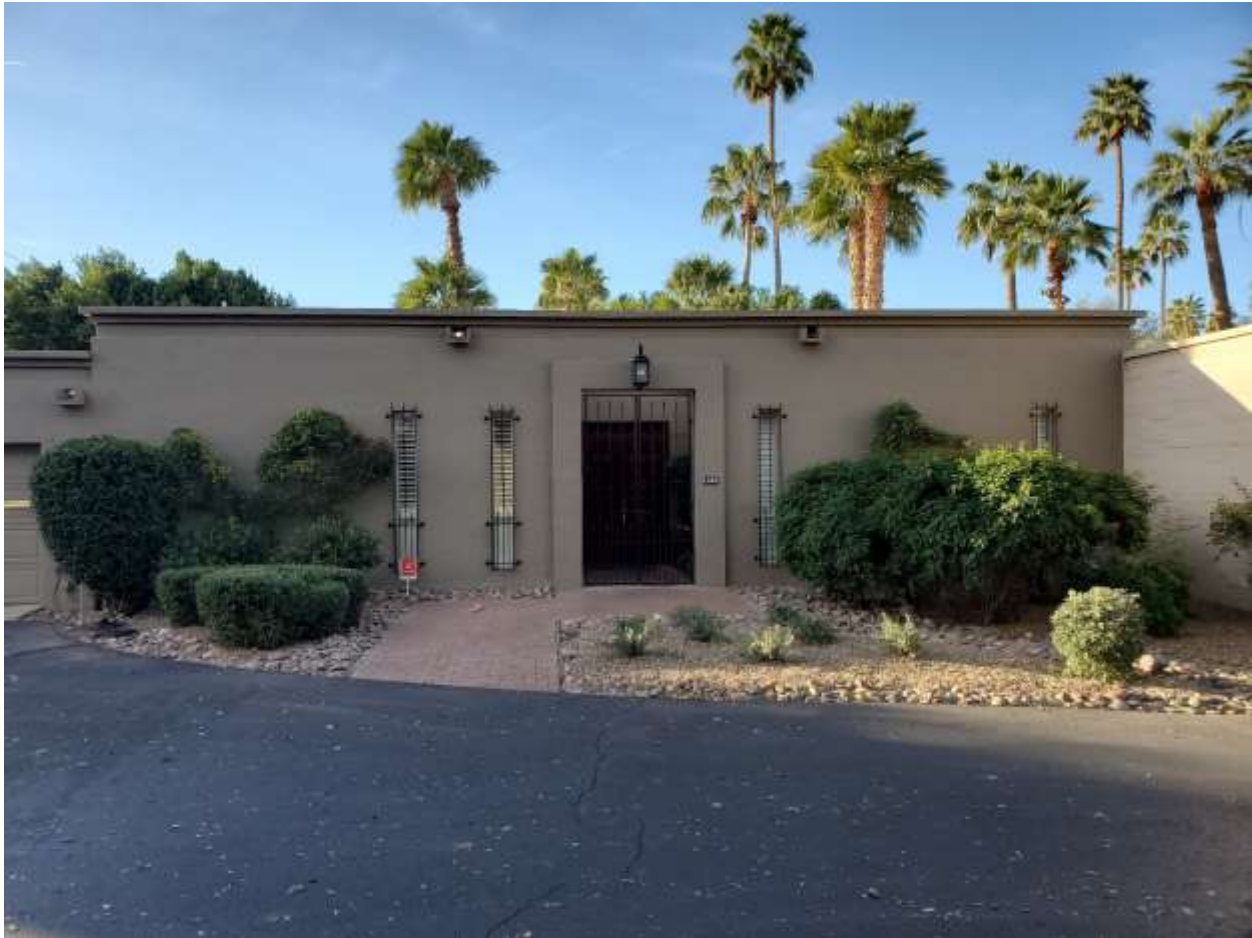
FIGURE 12 (NR Photo 3) Single story unit, with central entrance. Vertical windows exist on both sides of the façade. Wrought iron grates are original. The roofline is marked by a recessed band below a narrow molded cornice. The façade is has an original finish where the blocks are evident, but not pronounced.
