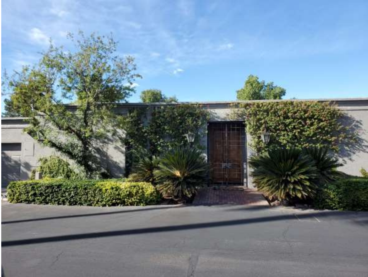
FIGURE 26 (NR Photo 17) Typical one story unit with original façade texture. The entry gates are replacements.
