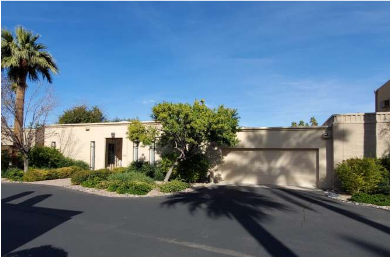
FIGURE 38 (NR Photo 29) One story unit with typical roofline detail, and deep recessed entry of 8 feet. The "fan/swirl" texture and pattern of the stucco is original.
